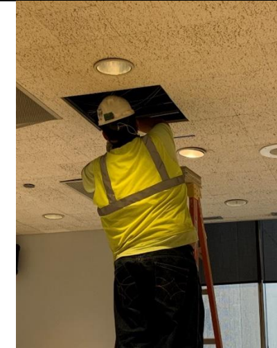
26MAY20: Contractors initiating work on HEPA Filter installation
